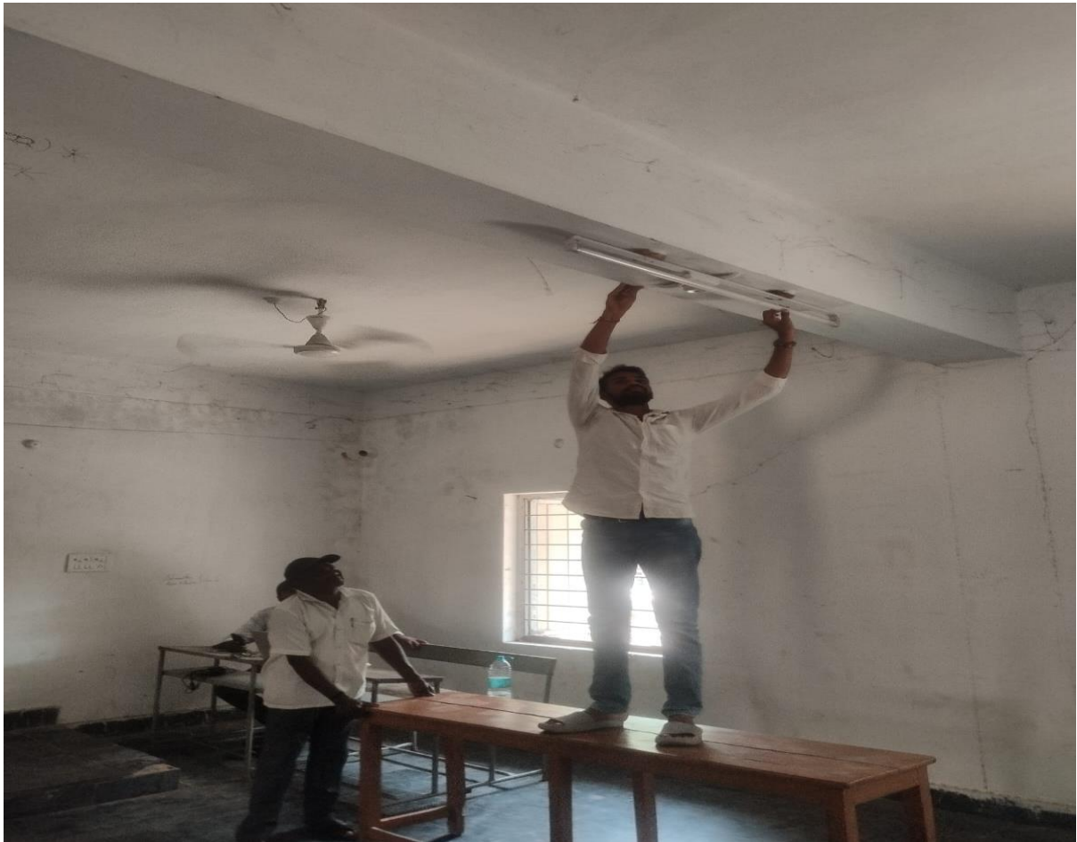
Installation of tube lights
